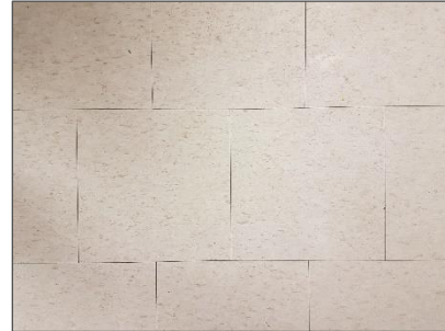
Non-asbestos, 12" x 12" brown splotch vinyl floor tile.
