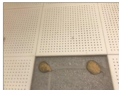
Non-asbestos, brown adhesive for wall mounted 12" x 12", glued-on, wood fibre tiles with pinholes.
