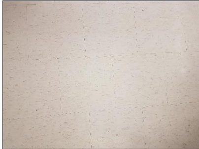
Non-asbestos, 12" x 12" white with grey splotch vinyl floor tile.
