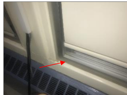
Non-asbestos grey caulking around windows.
