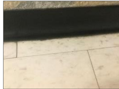
Baseboard with non-asbestos adhesive.
