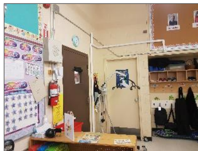
View of fibreglass insulation on pipes in Classroom 107.
